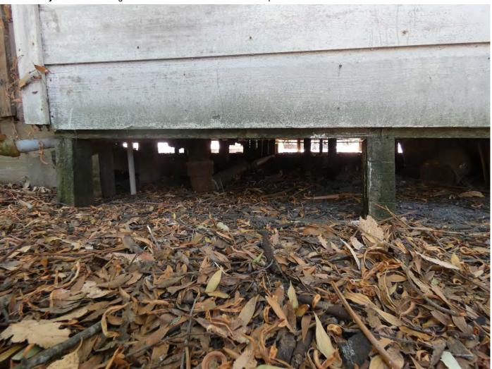
Figure 13 Residence. View to the South of beam-on-pier foundation. Photograph by Edward Yarbrough.
