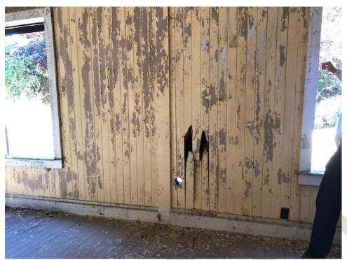
Photograph 37. Gas line stub (protruding from floor) and hole cut through wall, indicating possible gas fireplace within residence.
