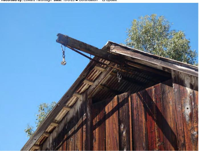
Figure 2 Barn's hoist beam. View to the West. Photograph by Edward Yarbrough.
